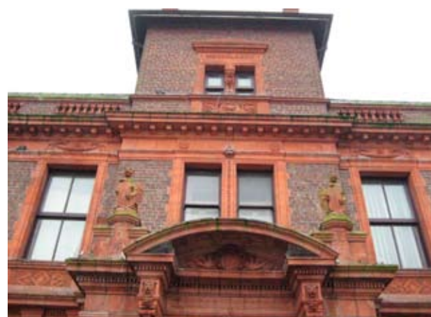
The old Town Hall, built 1885, is being converted to a hotel
