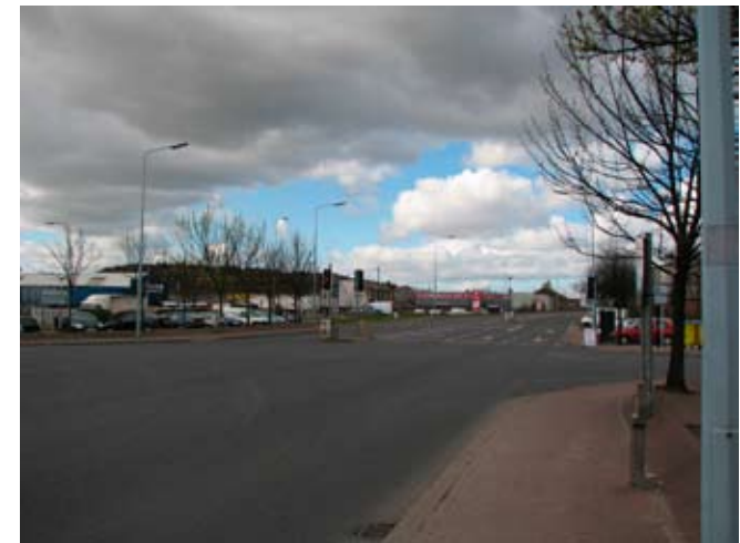
6.7 Junction of Ashley Way acts as a barrier to pedestrian movement south of Victoria Road
