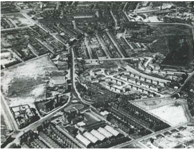
3.4 Inter-war aerial view showing the new Kingsway to the left.
