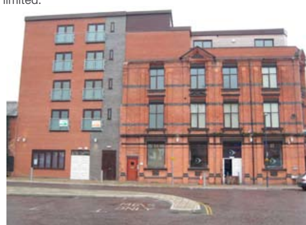
A combination of conversion and new build on Market Street.
